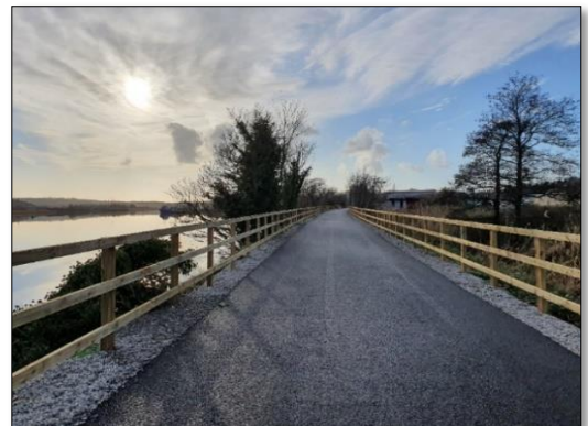
Image of completed section near Shanbogh New Ross with River Barrow vistas
