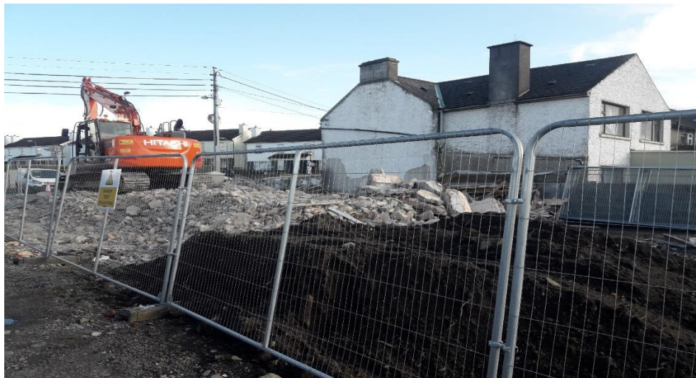
Demolition works at Golf Links Road Site
