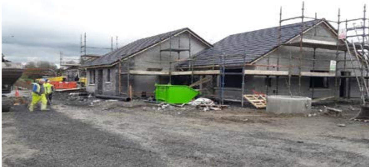
Works on Legan Grange, Thomastown ongoing
