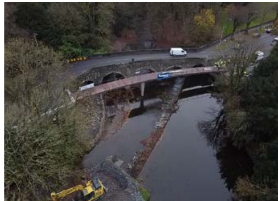
Drone view of new Footbridge and existing Road Bridge.
