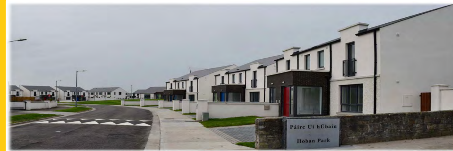
First Near Zero Energy Development in the entire Country at Hoban Park, Callan, Co. Kilkenny
