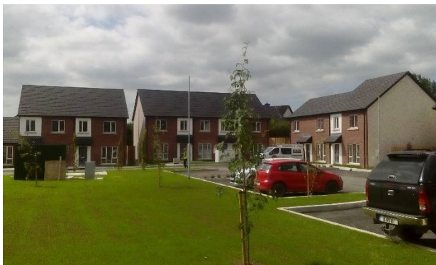
54 units Ballybough Street, Kilkenny - Respond Housing
